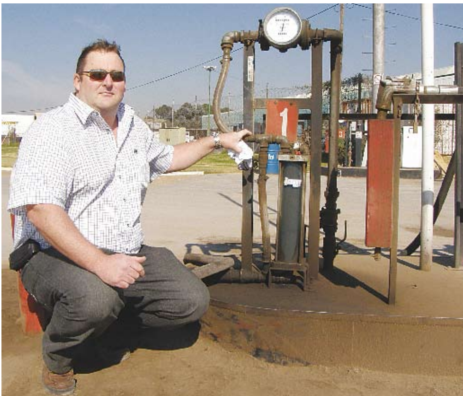
André Steyn of iFleet (Pty) Ltd, shows MechTech a ceramic diesel filter on trial at MacDonald Transport.
